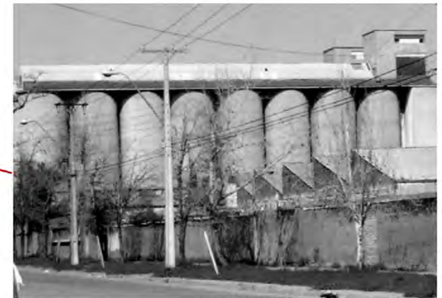
Ex ECA (demolida 2008)
