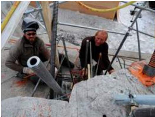
Fig 05.02 Montaje del anclaje a las rocas. [http://www.antarcticstation.org/assets/ceimg\\_cache/assets/uploads/modules\\_images/anchoring\\_650\\_366\\_80\\_s\\_c1\\_c\\_c.jpg](http://www.antarcticstation.org/assets/ceimg_cache/assets/uploads/modules_images/anchoring_650_366_80_s_c1_c_c.jpg)
