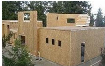
Fig. 19 (Casa en paneles SIP...Structural Insulated Panel )
